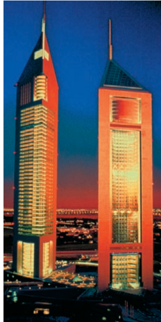
Emirates Tower Hotel in Dubai
