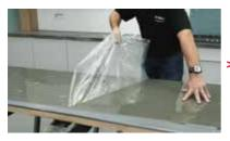
Remove the protective film from the BACK of the panel.
