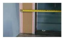
Measure between trims and mark on the back of the panel.
