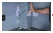
Dry fit the boxing, ensuring you use packers to check the fit.
