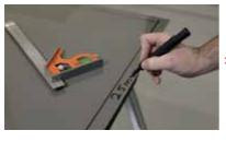
On the BACK, measure & mark 25mm line on all visible edges.
