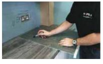
Using a marker pen, draw up the BACK edge of the boxing.
