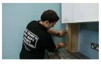
Place trims on the internal & external corners around the boxing.
