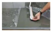
Peel off the double-sided tape & carefully apply the joining strip.
