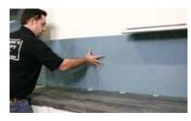
> Fit the panel to the wall, using packers for expansion.
