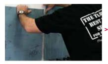
Slide that panel behind the other on the wall and remove tape to attach.
