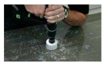
Use a holesaw to cut a hole through where the socket will sit.
